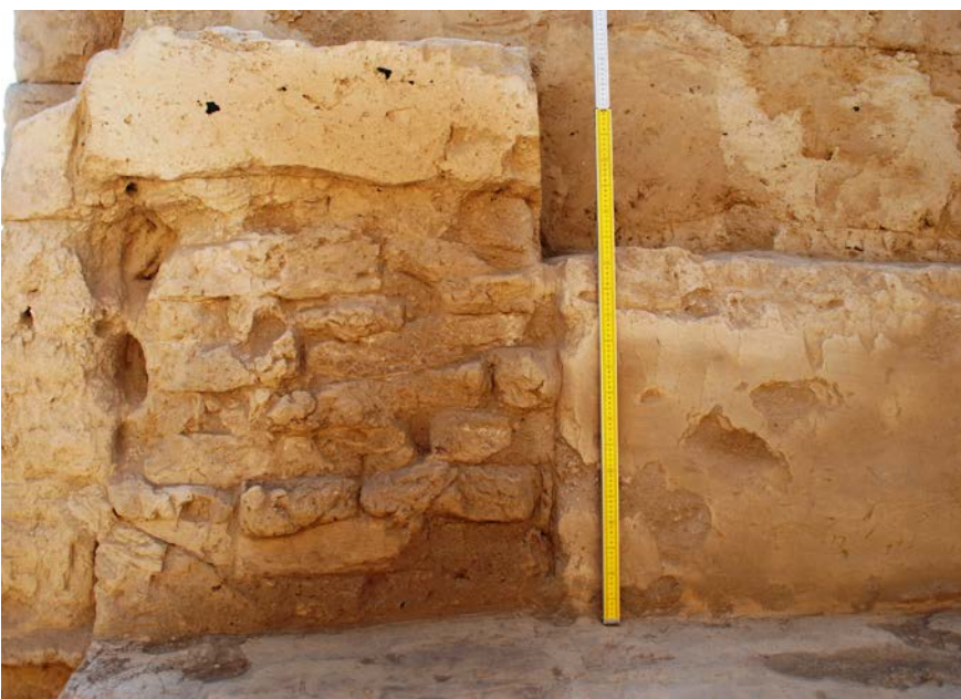
Fig. 27. The bricked-up entrance in eastern wall of Room No 1
